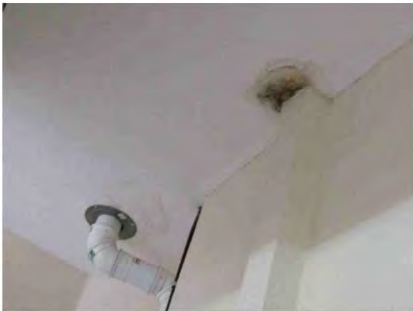
Black - mold like substance and water stain garage ceiling
