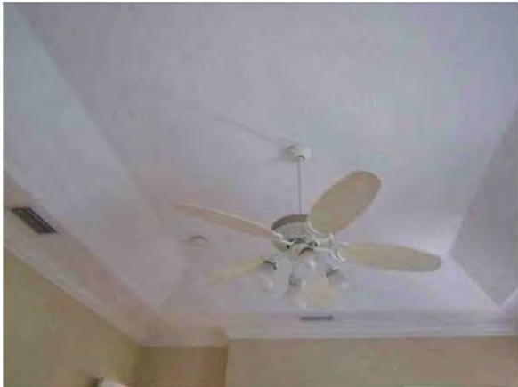
Tray ceiling Crown molding
